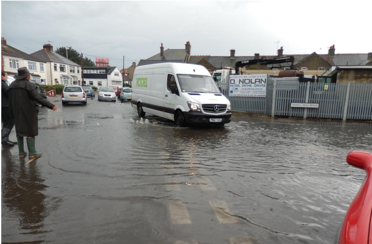
'Exceedance' of drainage capacity at A2 Canterbury Road, Sittingbourne where a large existing drainage system is present within an area of borough council owned green space. This flooding occurred in May 2019. A similar flood also occurred in August 2020 following a severe thunderstorm:
